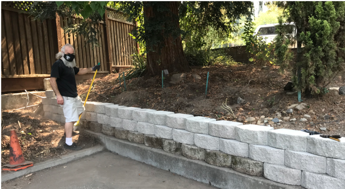
At September's UUFLG workday, member Ron Kirkland pauses from building a retaining wall.
